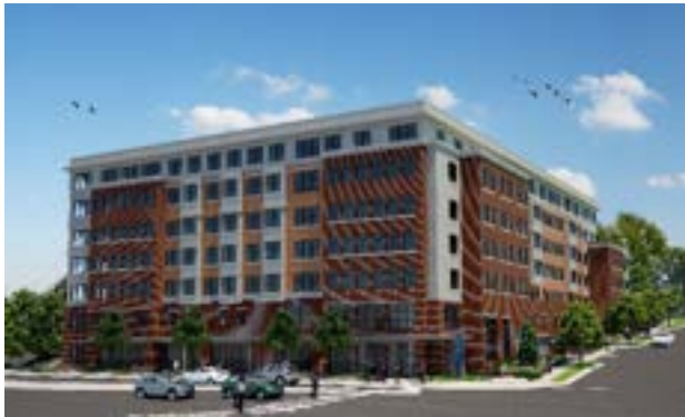
The Arden 126 units Alexandria, VA (Fairfax County)
